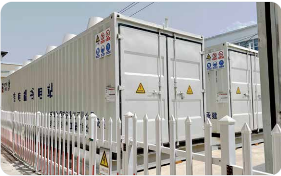
> 3MW/31MWh lead-carbon battery project (Changxing, Zhejiang, China)
