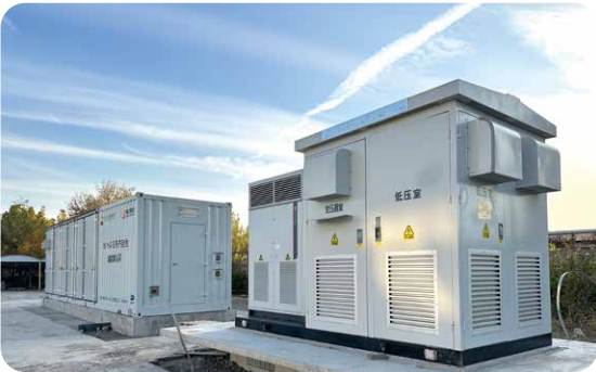
> Dagang oilfield 1MW/1MWh sodium-ion battery (Tianjin, China)
