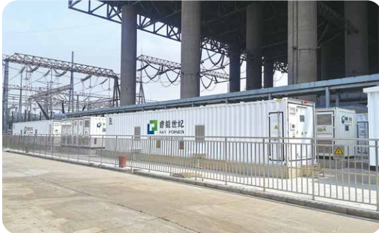
> 15MW/7.5MWh thermal power plant ESS (Shanxi, China)
