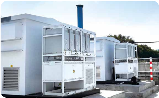
> 2MW PCS Skid (Qingyuan, Guangdong, China)
