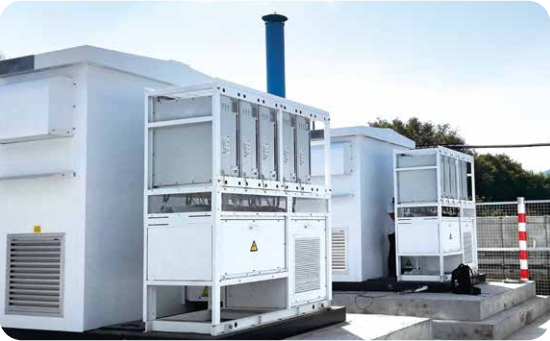
> 2MW PCS Skid (Qingyuan, Guangdong, China)
