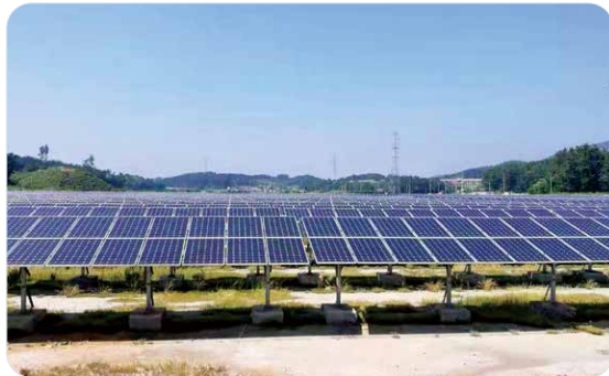
> South Korea 12MW/36MWh PV ESS (South Korea)
